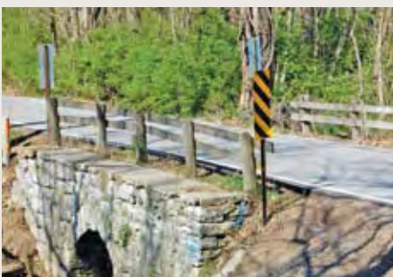
One-Lane bridge on Teson Road
