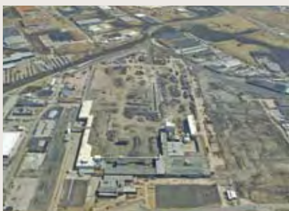
Aviator Business Park Demolition
